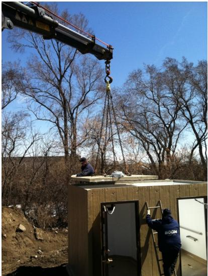
The green septic tape can be placed around the perimeter of the toilet body in preparation of the roof being set in place. The tape should be placed on the seam.
