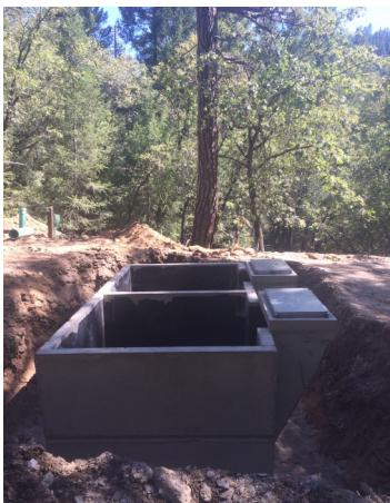
The body is set on the vault with the back and side walls flush with the vault. The septic tape will make a water tight seal.
